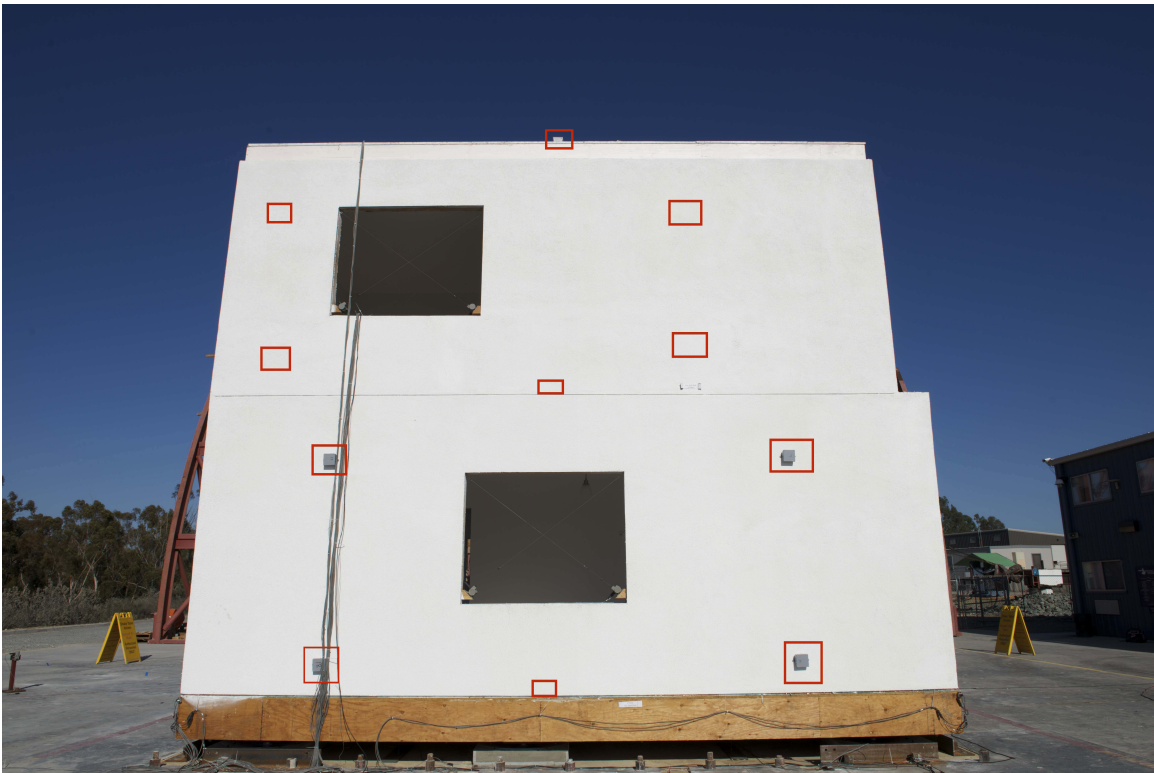
Figure 3: Sensor location on the West side wall: Exterior wall. The squares indicate the locations of the sensors
